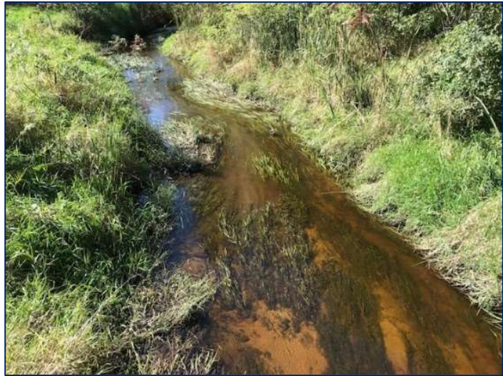
Figure 10- Branch & Derby Drain view from M-140 crossing looking downstream.
