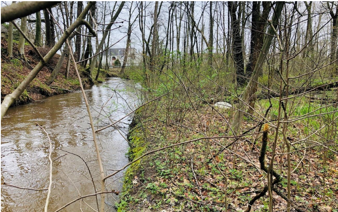
Figure 18 - Lower Branch & Derby Drain near outlet to Paw Paw Lake. Note that the drain is not connected to the floodplain at this location. Photo taken on April 29, 2020. Source: Spicer Group.
