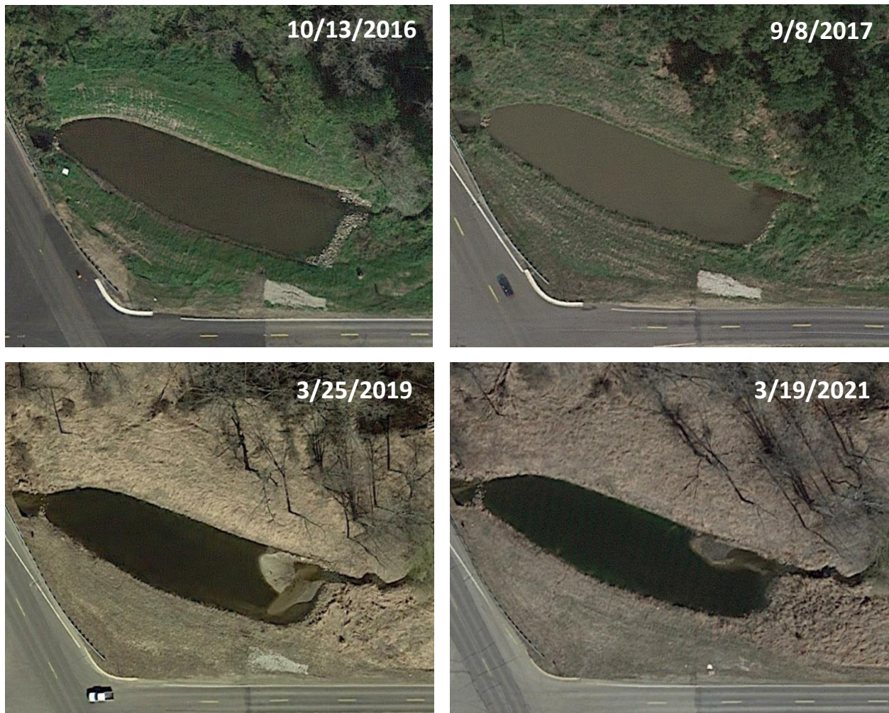
Figure 15 - Aerial view of the M-140 basin on the Branch & Derby Drain. Note the sediment deposition in 2019 and 2021 images.
